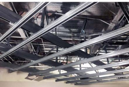
Unistrut metal framing is uniquely suited for state-of-the-art Cath Labs, distributing loads and prevents deflection for improved image quality. The support structure is discreetly hidden above ceiling panels, attached directly to structural elements like concrete decks or steel beams. Our customized design solutions meet weight requirements and equipment support needs within your budget and project timeline.
